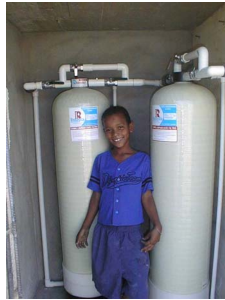
This chlorinating, activated carbon water filtration system will provide a consistent supply of clean water to the orphanage in Esperanza for the first time.
