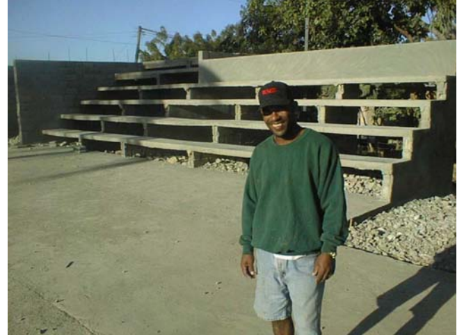
The bleachers in Esperanza were completed. People will use the bleachers to watch games and programs.
